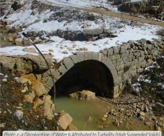
Photo 4 - 4 Discoloration of Water Is Attributed to Turbidity (High Suspended Solids)
