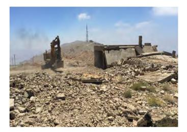
Photos 5-28 Demolished Concrete Structures
